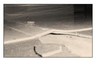
severe compression. Slab shrinkage can also lead to cracks. At times, these cracks can reflect through installed tiles. Control joints placed in the concrete to relieve the shrinkage can also reflect cracks through tiles. Tile pattern layout and movement joint details should be addressed to accommodate these joints or use products to help isolate the joint from affecting the tile.
