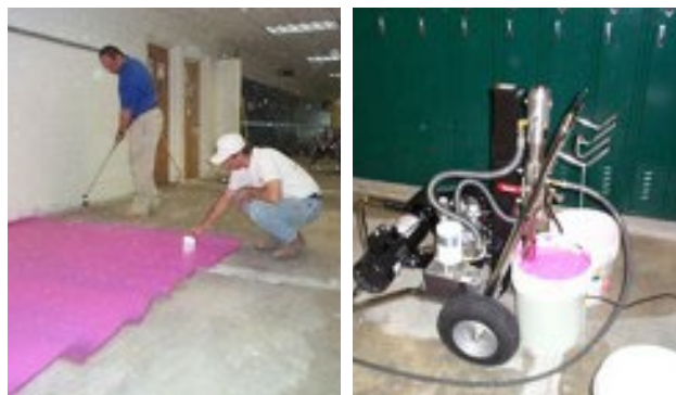
Checking thickness with a wet film gauge
