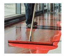
**TechLevel<sup>TM</sup> XP-1** is an innovative, high performance formula for demanding applications, especially where heavy rolling loads are anticipated. With a compressive strength of 5500 psi, Techlevel XP-1 supports the highest point load of any CustomTech SLU. Techlevel XP-1 provides a durable wear surface for construction traffic; however, it is not recommended as a long-term wear surface. Additionally, this product contains the low prep feature.
