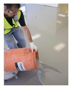
SLUs are slow to dry and will significantly delay the flooring installation. Furthermore, gypsum SLUs are only suitable for dry areas and cannot be used where standing water might be anticipated. Gypsum SLUs are less resistant to damage from trade traffic.
