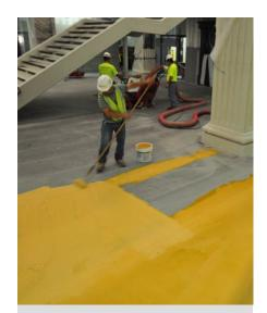
The performance of the membrane is dependent on correct, continuous coverage.
