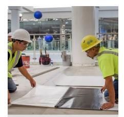
There are many reasons for using a membrane in a ceramic or stone tile project. Membranes are commonly used to prevent cracks in the substrate from migrating into the tile.
