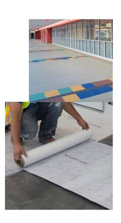
The performance of the membrane is dependent on correct, continuous coverage, and if the application is too thin, it may fail. Brushing, rolling and spraying can leave voids or pinholes in the film that will allow water to penetrate to the substrate. If waterproofing is the goal, a second coat must be applied to ensure that all voids are filled before installing tile.
