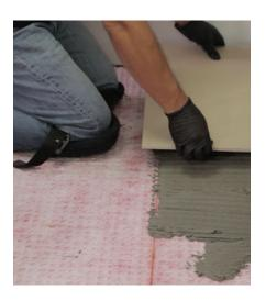
It is easier to predict the time required to install tile when using a cement mortar-bonded sheet membrane. The curing process of the cement mortar doesn't rely on the primer drying. Since the cement mortar remains workable for some time, these membranes can be easily repositioned if required. Peel-and-stick membranes are usually not repositionable. This makes it critical that the peel-and-stick membrane is placed properly the first time.
