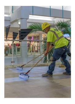
An increasing number of membranes fulfill more than one role in the tile assembly. This paper will explore the uses for these versatile, multipurpose membranes.
