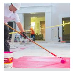
Some membranes provide a waterproofing barrier in addition to crack isolation.
