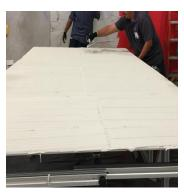
Apply mortar to both the surface of the substrate and the back of the tile/panel. The trowel ridge lines should be applied to these surfaces so they are parallel to the short side of the panel/slab and to each other when pressed into place. This will prevent trapping air under the tile and creating a void.
