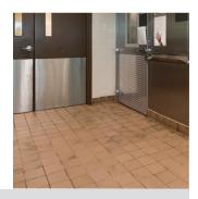
Build up of grease and fatty acids will disintegrate grout.
