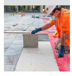
also provides a solid base as voids may allow a collection of water, leading to freeze-thaw damage. (Back-buttering the tile alone does not constitute coverage; mortar needs to make full contact with tile and substrate. Back buttering tile is highly recommended for all exterior installations.)
