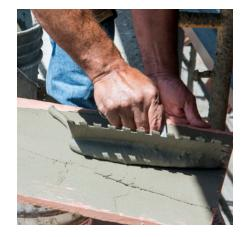
Back-buttering the tile alone does not constitute coverage; mortar needs
