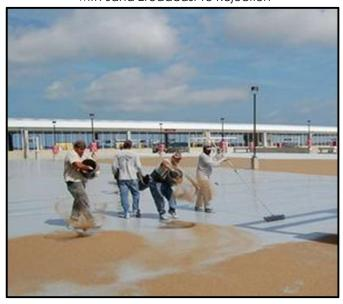
Once the excess sand is removed, the options for assemblies are similar to the traditional TCNA thinset method (F104) and thickset bonded mortar bed method (F101).
