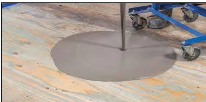
Self-leveling underlayment over plywood
