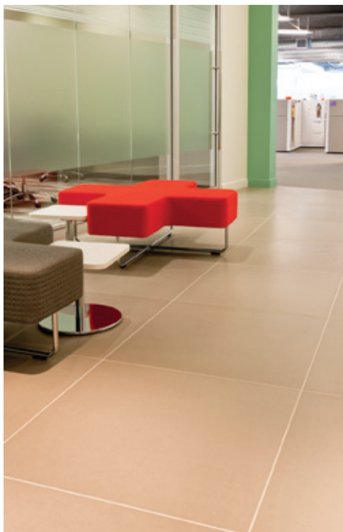
3' x 3' Installed Porcelain Tile Brocade Communications Systems, Inc., San Jose, CA
