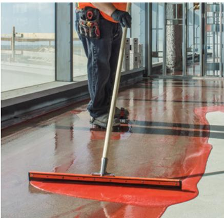
Floor prep began with shotblasting, followed by a coat of CustomTech<sup>®</sup> TechMVC<sup>™</sup> Moisture Vapor and Alkalinity Barrier. TechMVC is a high-density, 100% solids epoxy that can be used on concrete measuring up to 100% R.H., 25 lbs. MVT and pH 14 to bring floors into compliance with ASTM F-710. Single-coat application effectively controls concrete moisture emission and creates an alkaline barrier between the substrate and moisture-sensitive adhered flooring materials.
