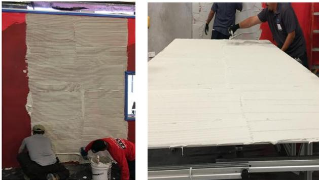
Apply mortar to both the surface of the substrate and the back of the tile/panel. The trowel ridge lines should be applied to these surfaces so they are parallel to the short side of the panel/slab and to each other when pressed into place. This will prevent trapping air under the tile and creating a void.
