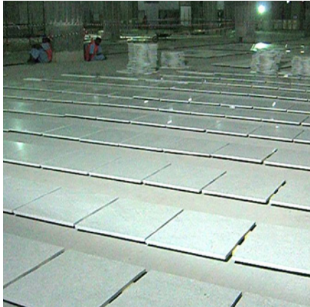
Photo 5: Insuring Tiles are Staged for Proper Sealing and Cure
