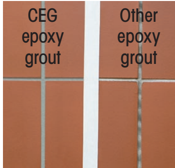
NON-SAG: Grout stays where you put it.
