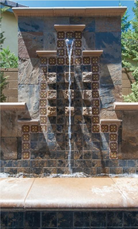
Be sure to select a grout type and color that is suitable for submerged conditions. CUSTOM Prism® color consistent grout holds up well to the water chemistry found in most pools today.
