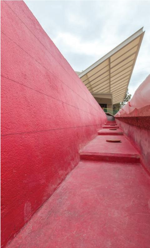
RedGard® Waterproofing and Crack Isolation Membrane is a liquid formula that is easy to apply to the unique curves found in many swimming pools.
