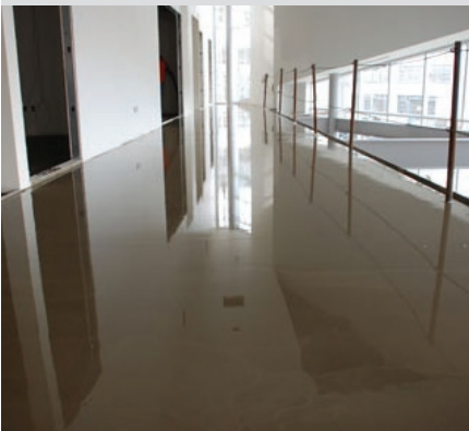
Photo Courtesy ABW Construction – Woodinville, WA
