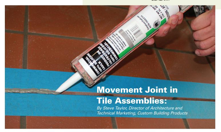
There has been considerable discussion concerning the need for movement joints in tile assemblies. The question is not whether they are needed; that is a simple yes. The questions are "Where do they go?", and "What is used to fill the joint in the tile assembly that will control or compensate for movement in the entire assembly?" There are several different types of construction movement joints defined by the Tile Council of North America (TCNA) that are needed in tile assemblies:
