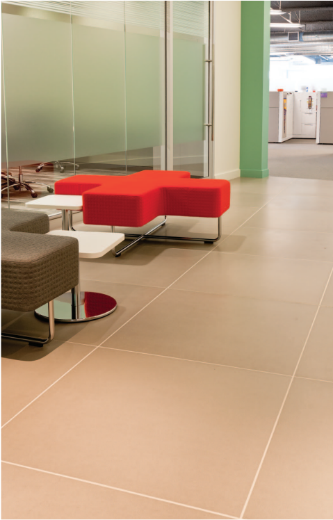
3 Foot x 3 Foot Installed Porcelain Tile Brocade Communications Systems, Inc., San Jose, CA
