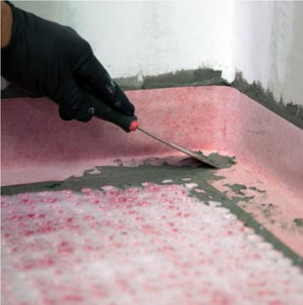
**Properly installed membranes extend the life expectancy of the tile installation.**
